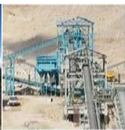
Copper Process Plant
