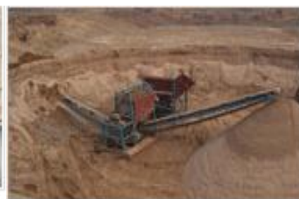
Stannum Process Plant
